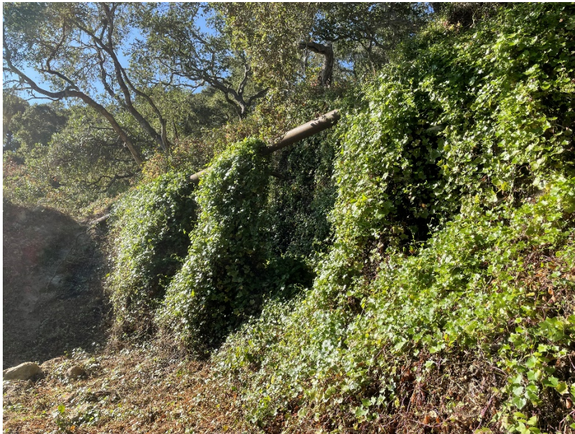
Figure 2: Pipe on Supports
