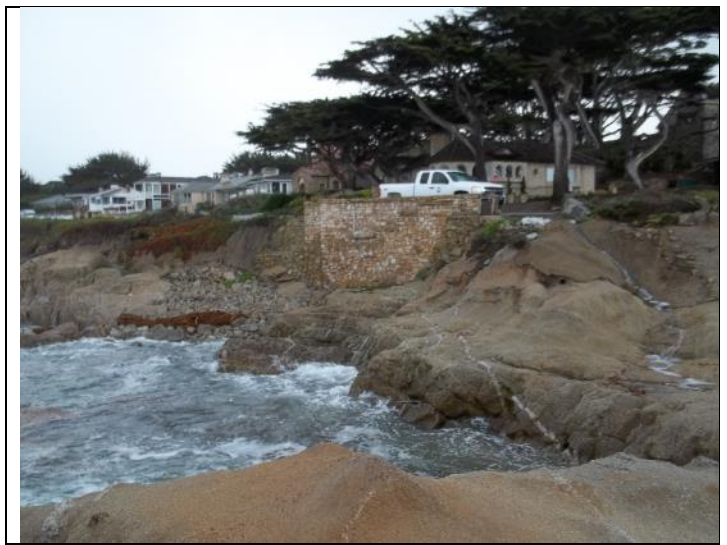
Photo: Looking at Pump Station Exterior
