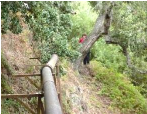
Photo: View gravity pipe in Carmel easement
