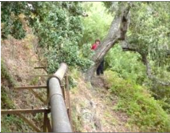
Photo: View gravity pipe in Carmel easement
