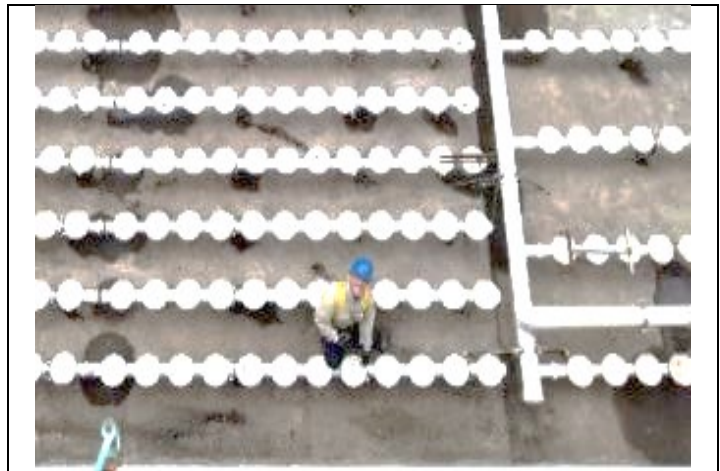
Photo: Existing air diffuser system
