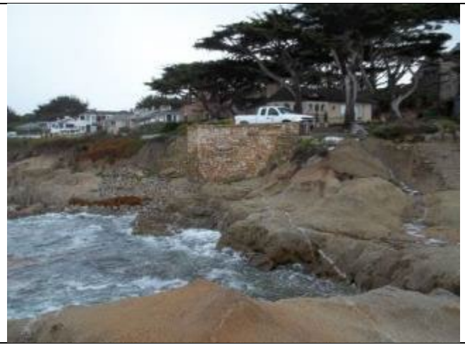
Photo: Looking at Pump Station Exterior
