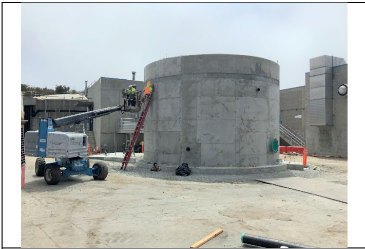
Photo: New Sludge Tank Under Construction
