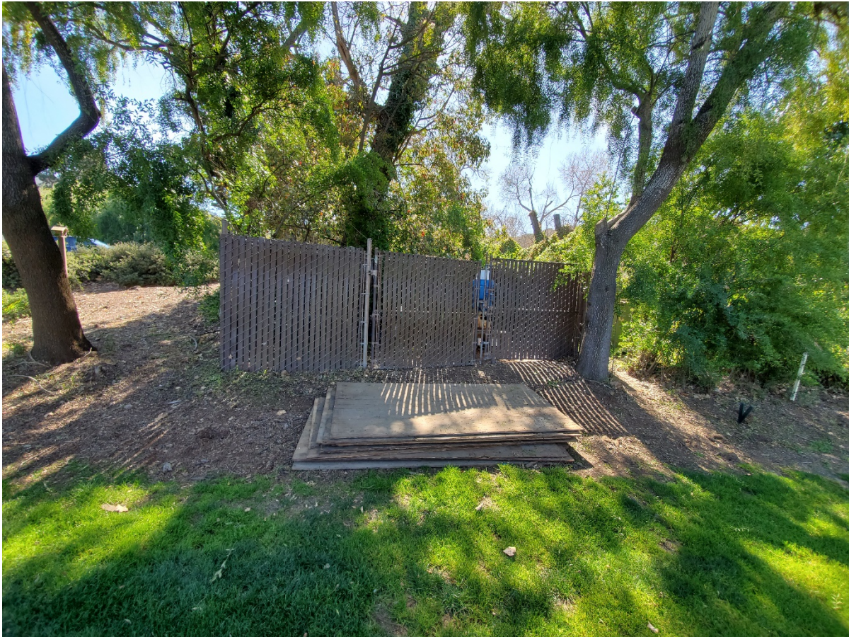
Figure 5 View of Similar Utilities Infrastructure near the Golf Course
