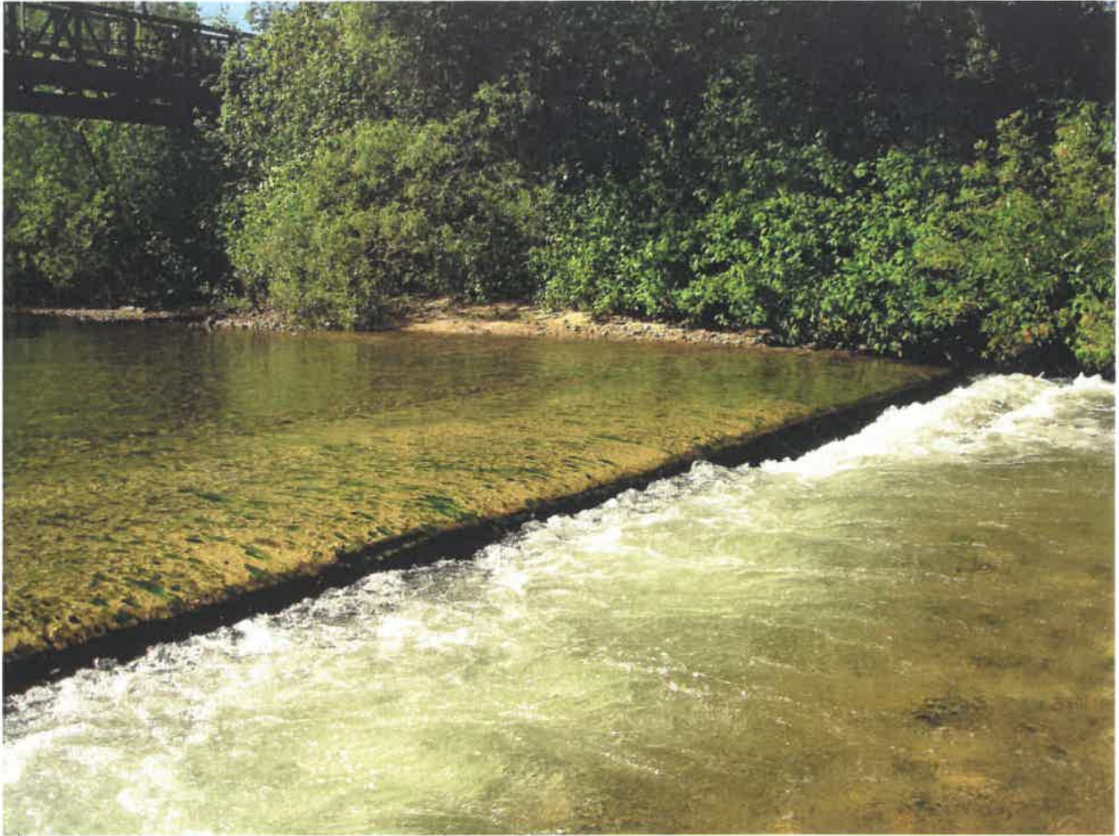
CAWD pipe crossing under Carmel River
