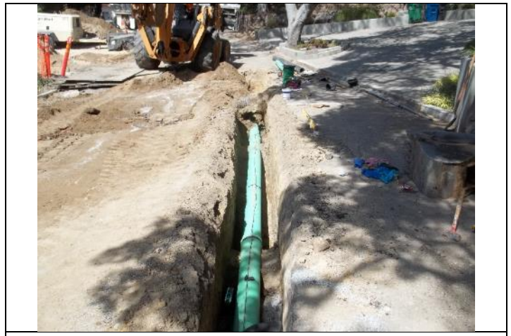
Photo: Sewer Line Repair
