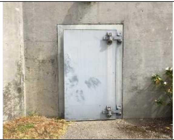
Photo: Old Flood Door in Headworks Basement
