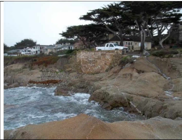
Photo: Looking at Pump Station Exterior
