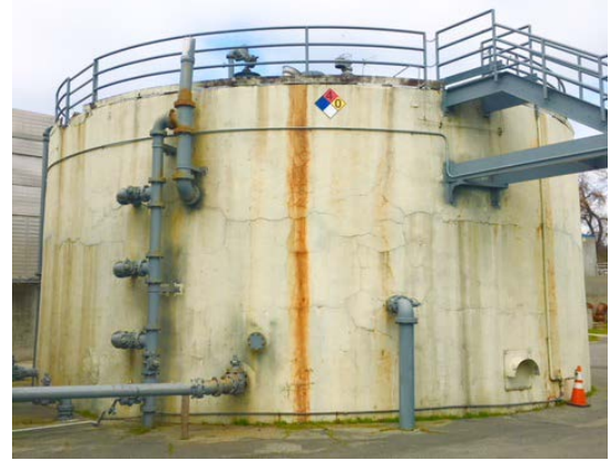
Photo: Old Digester No. 2
