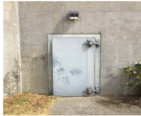
Photo: Old Flood Door in Headworks Basement
