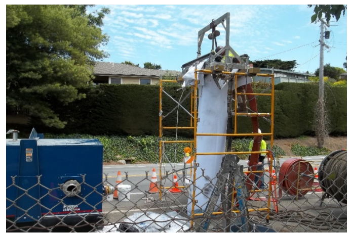
Photo: View CIPP Liner being installed
