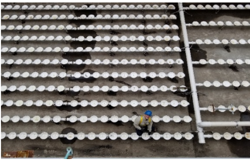
Photo: Existing air diffuser system
