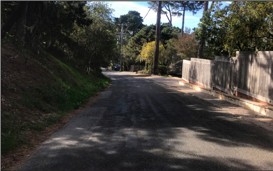
Photo #7: Pipeline alignment from Corona Road.
