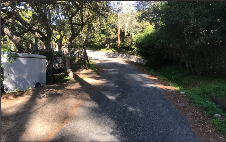
Photo #3: Pipeline alignment from Corona Way.
