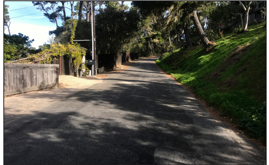
Photo #8: Pipeline alignment from Corona Road.
