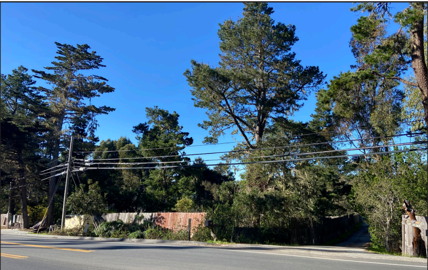
Photo #11: Location of Pump Station on the west side of State Route 1.
