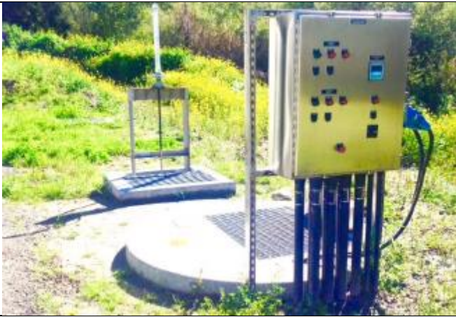
Photo: WWTP Stormwater Pump Station
