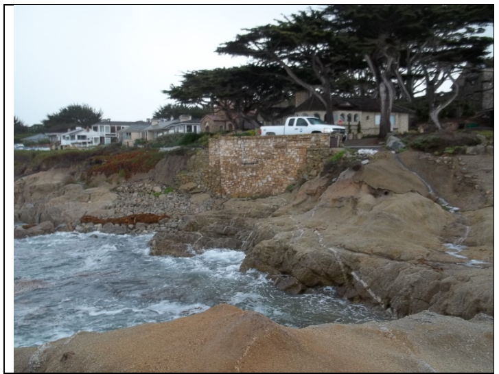
Photo: Looking at Pump Station Exterior
