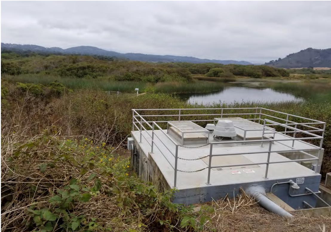
Figure ). View of Project Area from Calle la Cruz Pump station.
