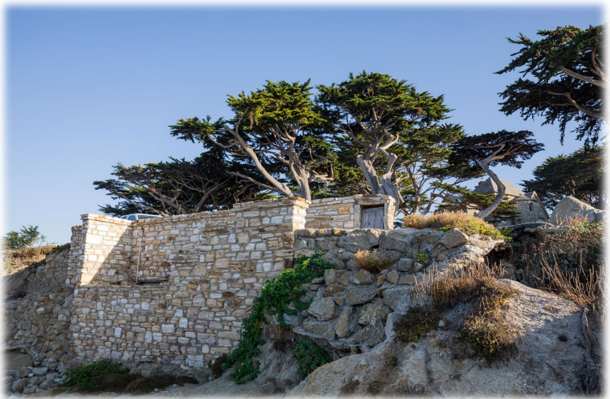
Bay & Scenic Pump Station
