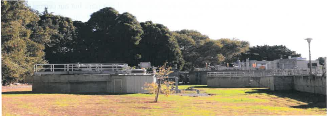
Clarifiers tanks & DAFT
