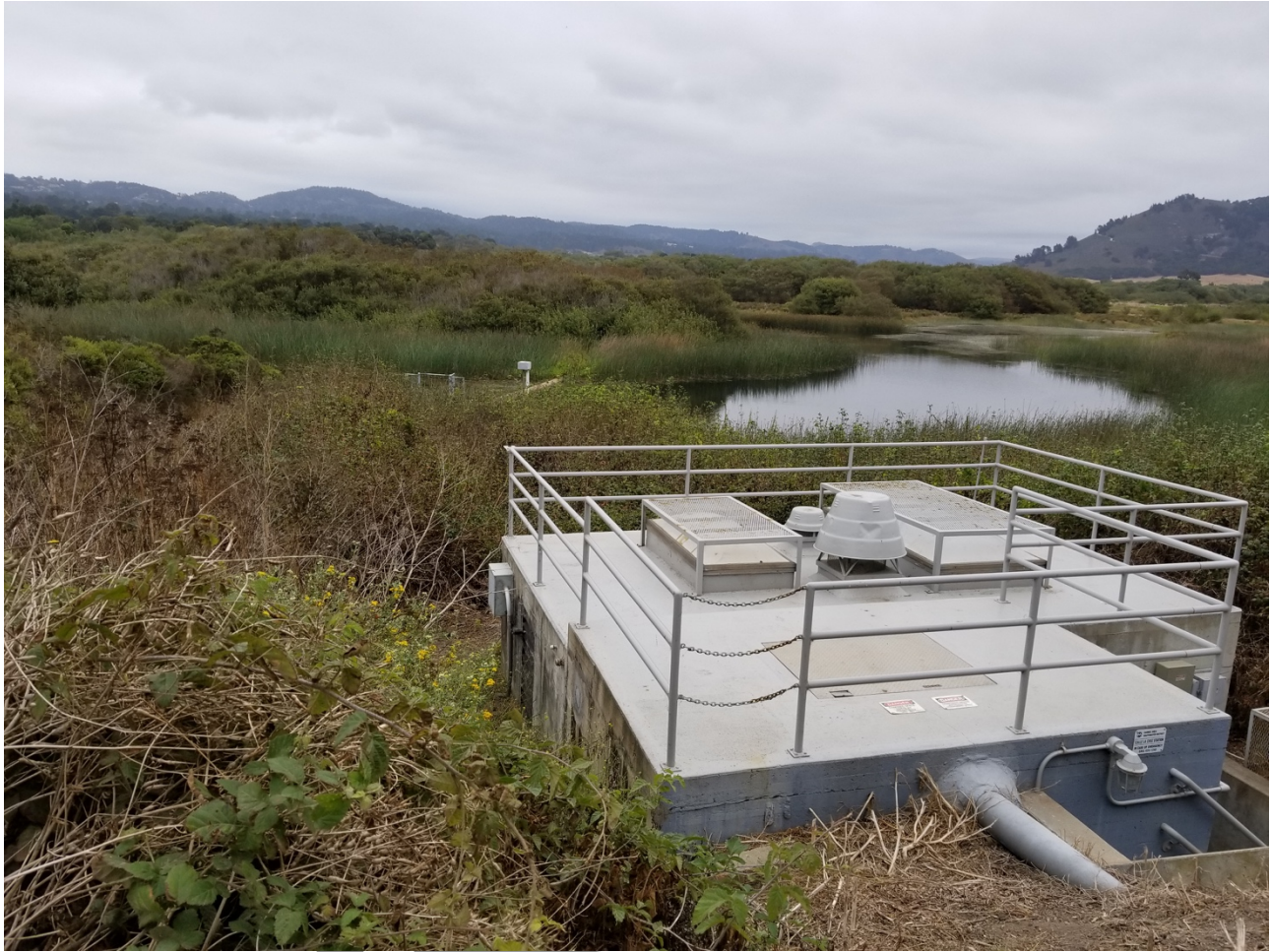
Figure 5. View of Project Area from Calle la Cruz Pump station.
