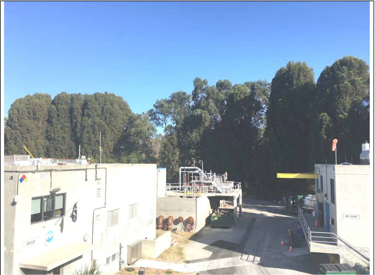
Photo 8: Taken from on top of an existing building inside the WWTP looking North at Northern property line. Note gap in eucalyptus filled in with cottonwood trees.
