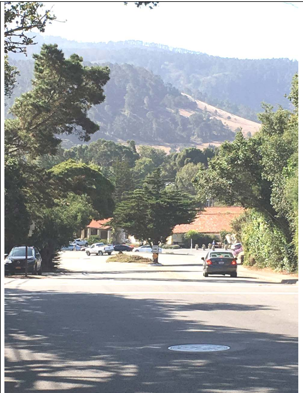
Photo 10: Taken from Rio Rd at Santa Lucia Ave Looking South at the WWTP.
