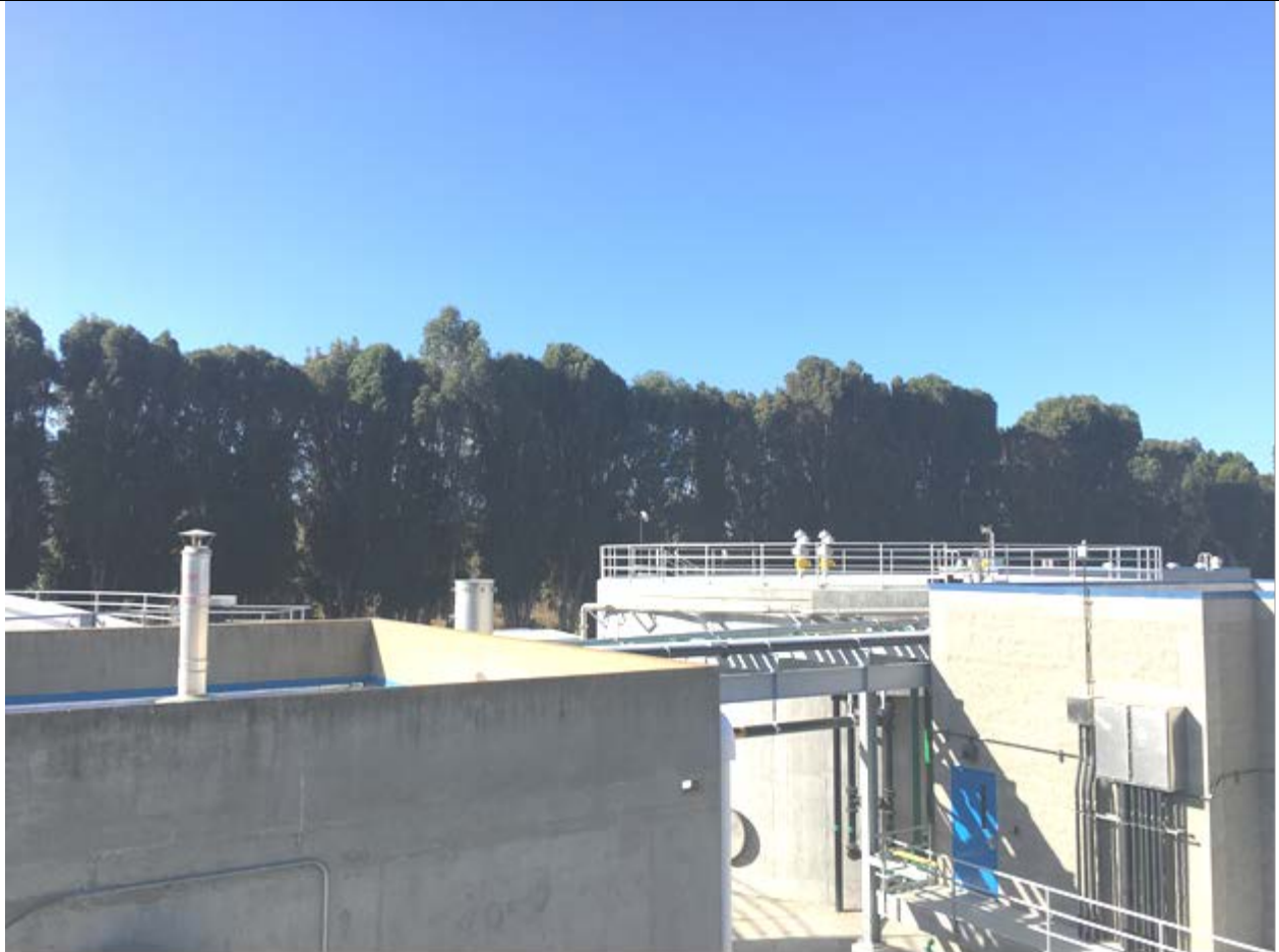
Photo 2: Taken from on top of an existing building inside the WWTP looking Southwesterly at southern property line.
