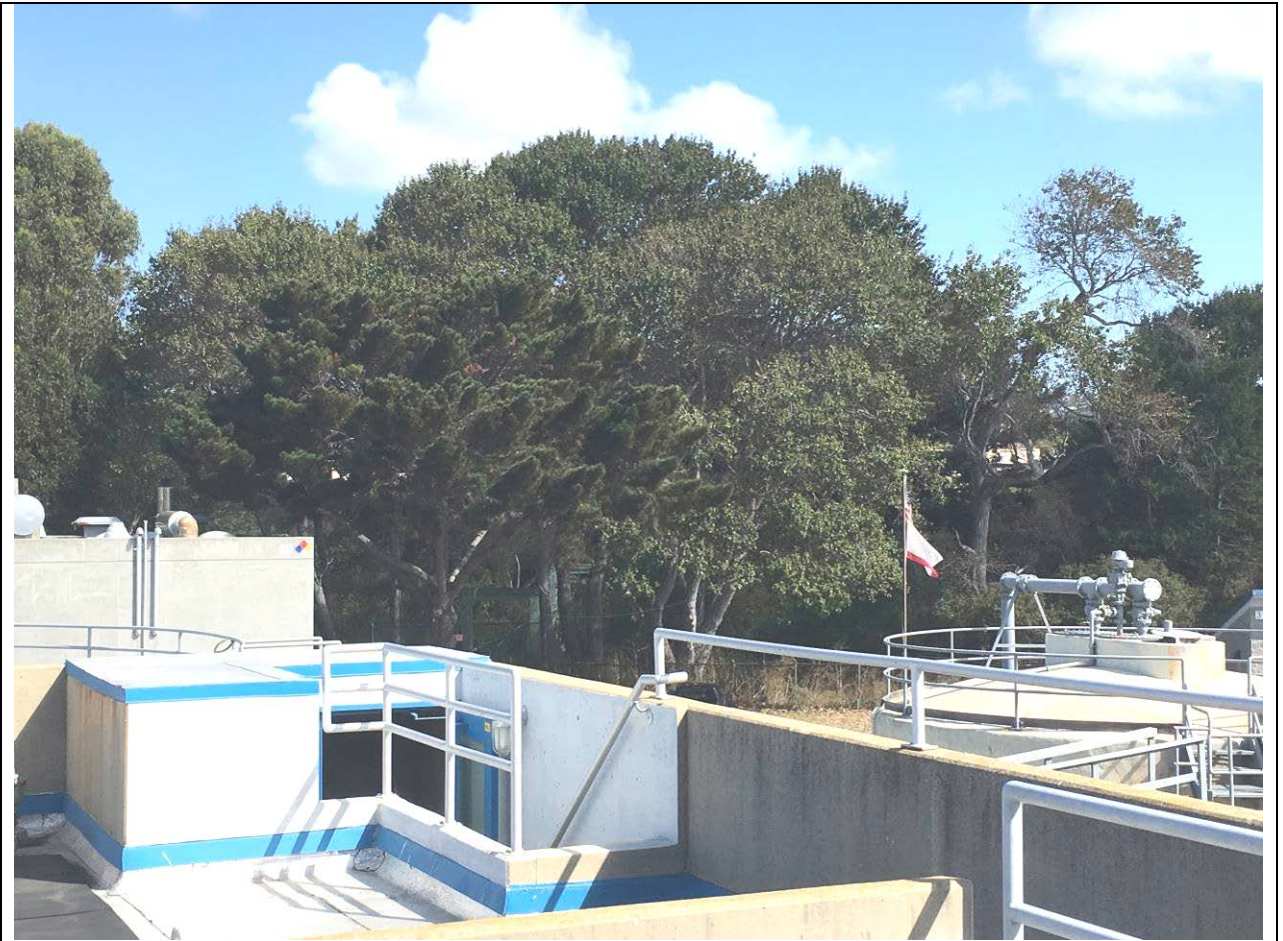
Photo 9: Taken from on top of an existing building inside the WWTP looking Northeasterly at Northern property line (No Eucalyptus). Note that buildings can be seen in the distance through gaps in the existing cottonwood trees.
