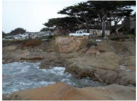
Photo: Looking at Pump Station Exterior
