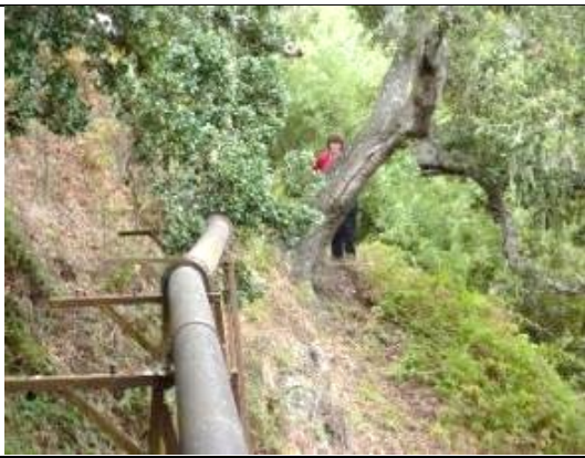
Photo: View gravity pipe in Carmel easement
