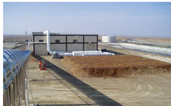
South Kern Compost Manufacturing Facility. Synagro utilizes an enclosed biosolids receiving and mixing building along with biofiltration in its compost system that controls VOCs and odors for the surrounding area.
