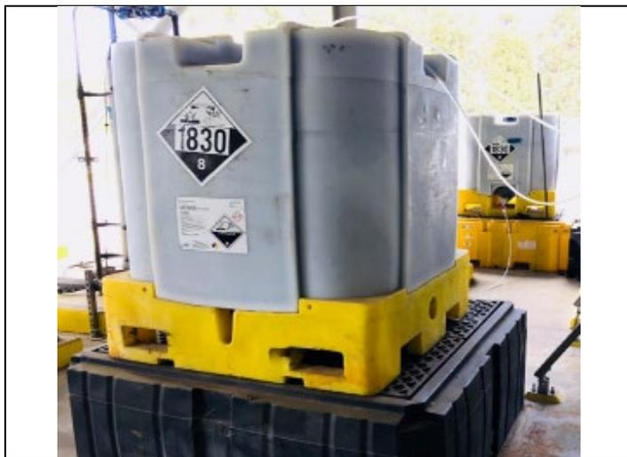
Photo: Existing totes used for Sulfuric Acid storage and Feed
