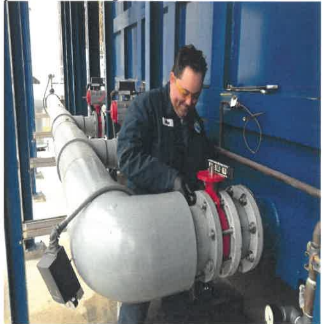
Repairs at Reclamation
