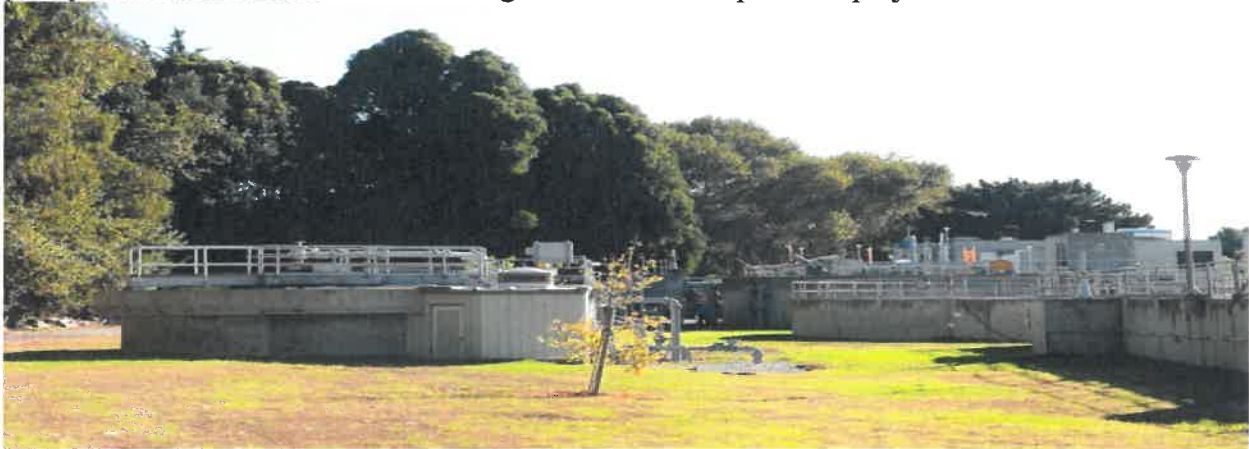
Clarifiers tanks & DAFT
