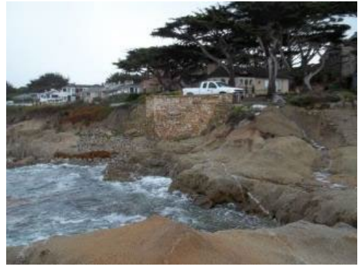
Photo: Looking at Pump Station Exterior
