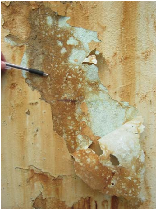
Figure 3: Rust Stain coming out from the Wall
