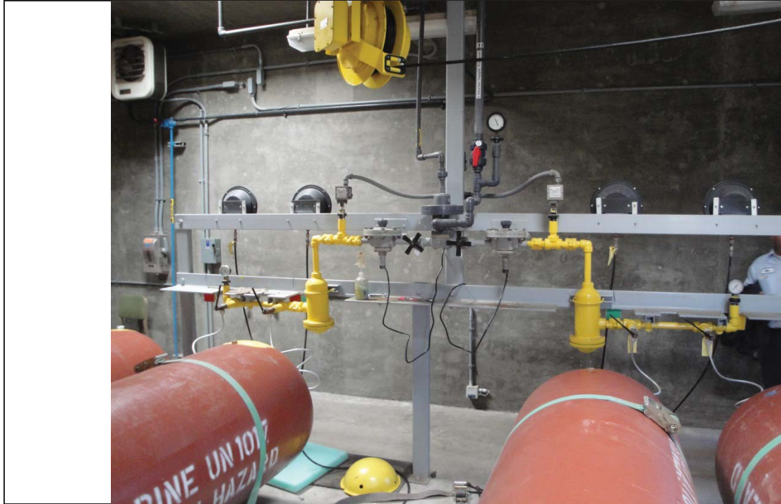
Chlorine Gas Feed Header with Automatic Shutoff Valves
