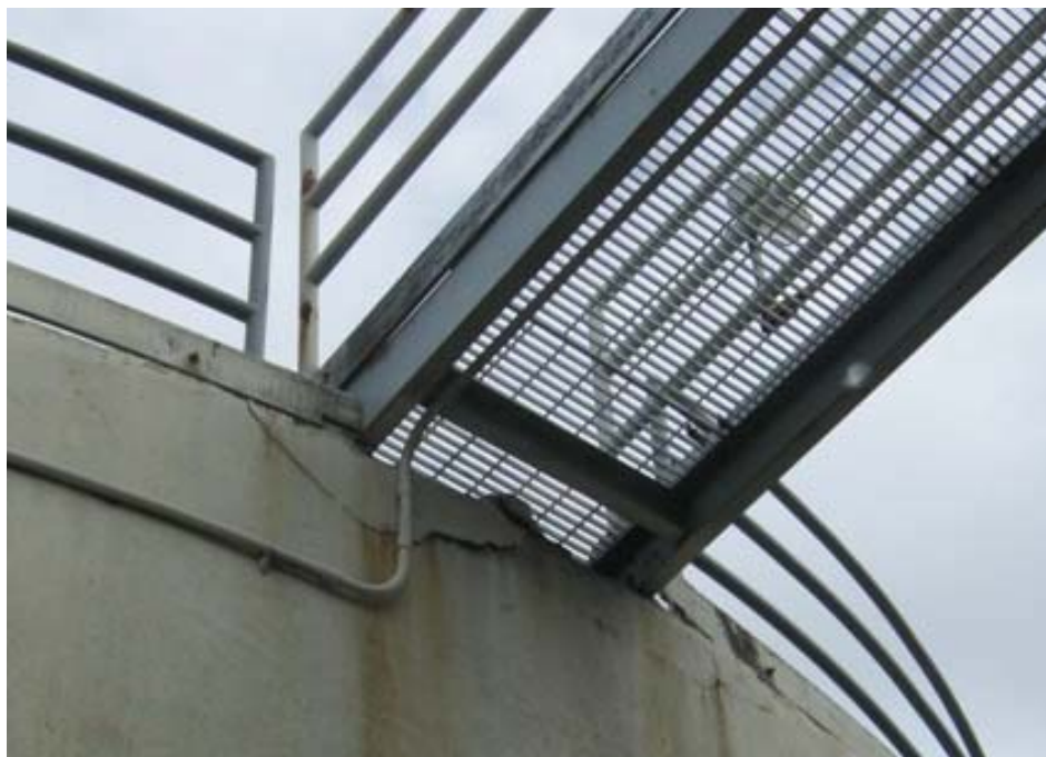
Figure 6: Spalled Concrete at Walkway Connection
