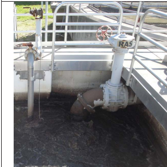
Corroded RAS Piping
