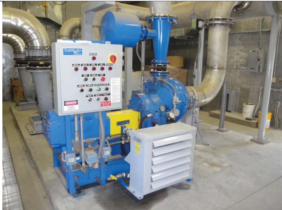
Only Reliable Aeration Blower (Turblex)
