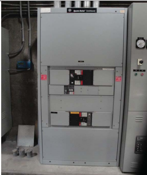
Distribution Switchboard "ISD2" (Blower Building, Main)
