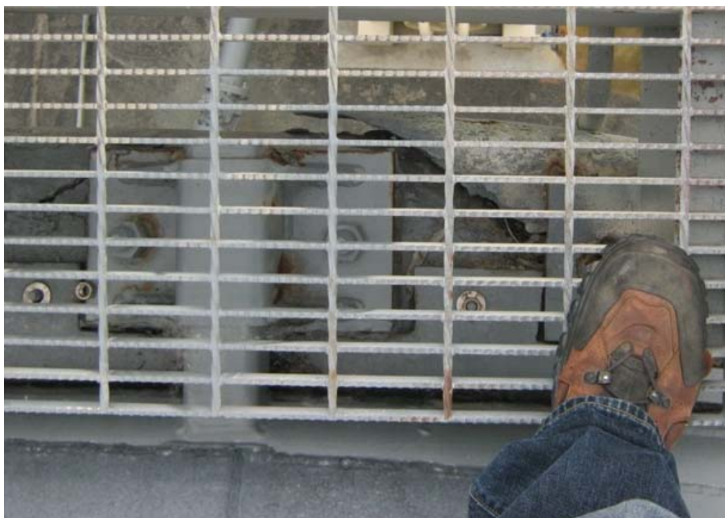
Figure 7: Cracked Concrete at Walkway Connection (Top View)
