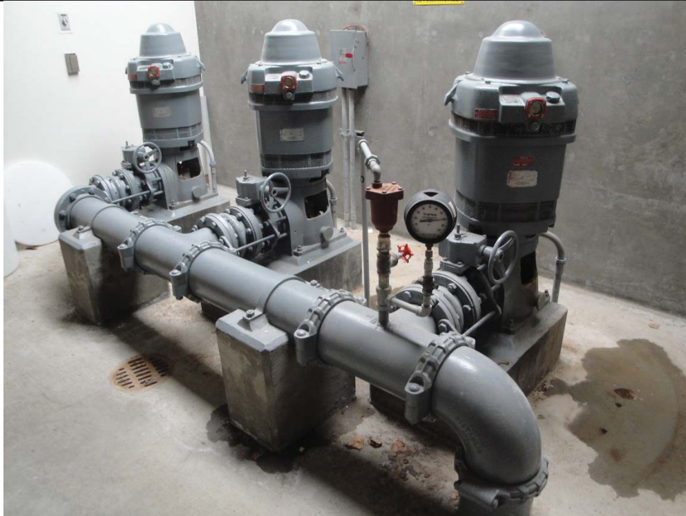
3 Water Supply Pumps
