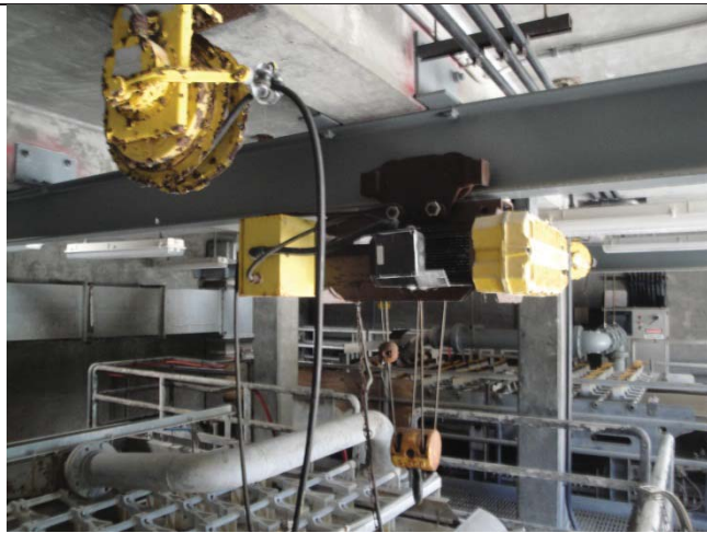
Severely Rusted Monorail Crane Equipment
