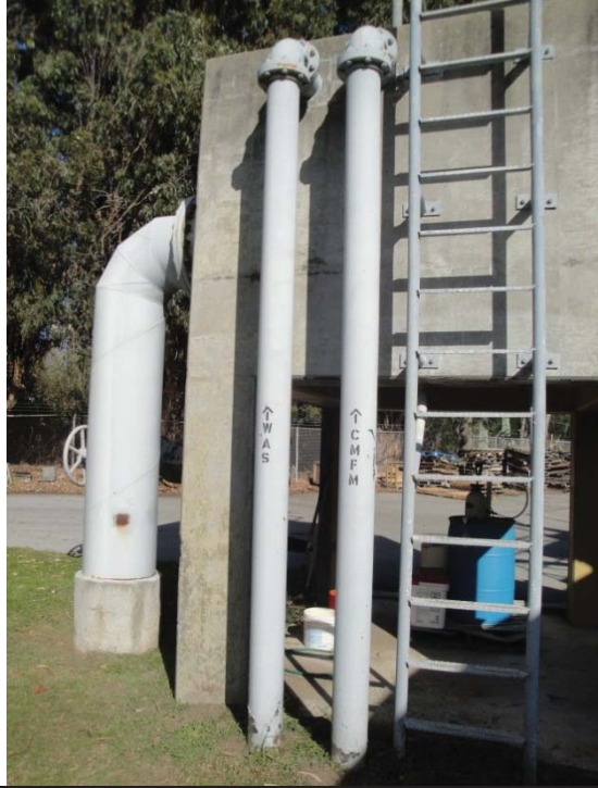
Piping Into Influent Manhole
