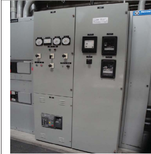
Generator Switchgear built in 1982
