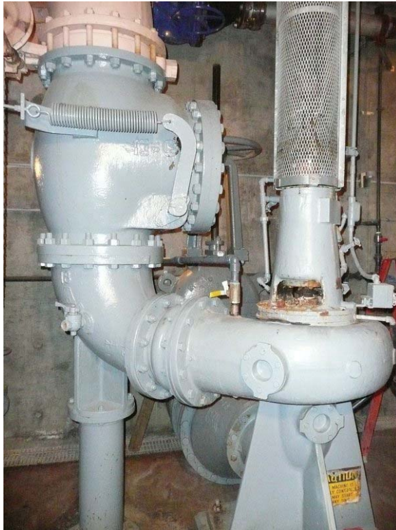
Figure 4: High-Service Pumps
