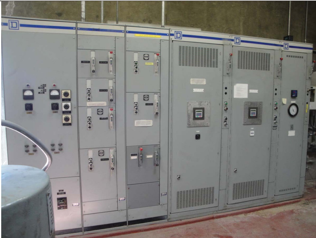
Effluent Building Electrical Gear
