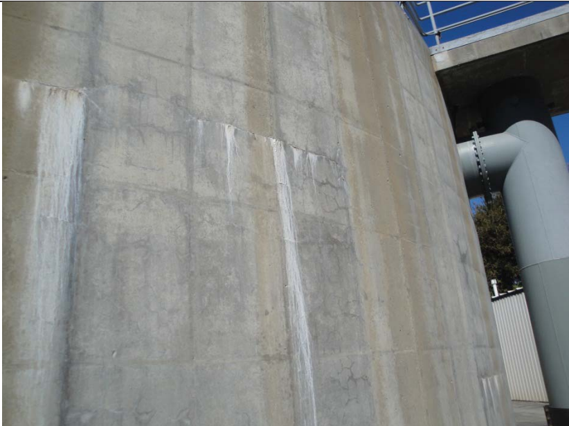
Digester 1 Concrete Horizontal Crack
