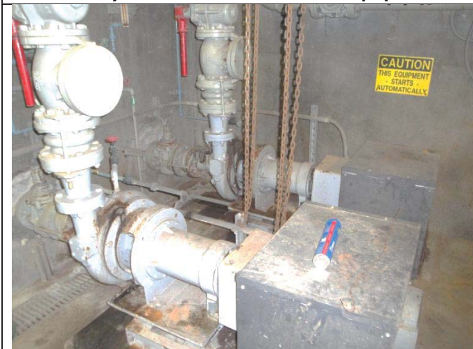
Filtrate Return Pumps
