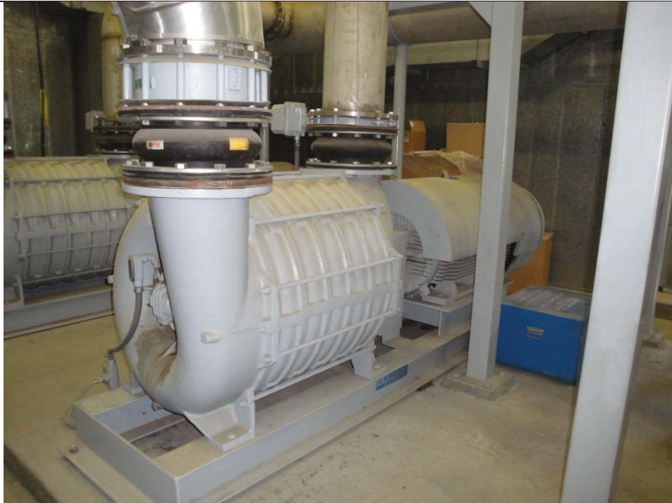
Oversized Standby Blower with Bent Shaft
