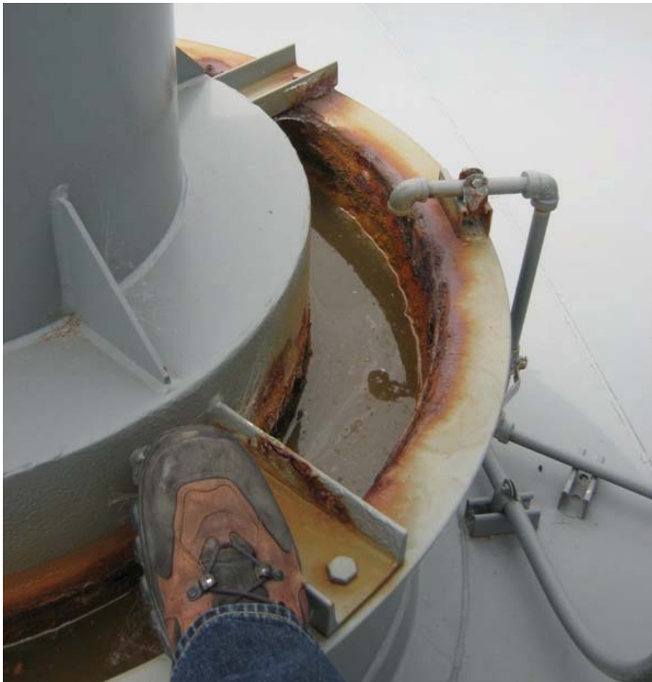
Figure 4: Rusted Water Seal on Cover
