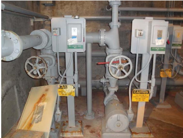
Figure 5: Treated Water (No. 3 Water) Pumps
