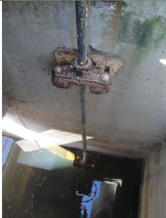
Corroded Sluice Gate Stem Operator Guide
