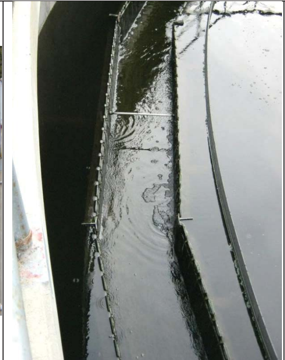
Secondary Clarifier Effluent Launderer
