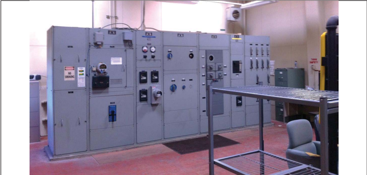
Main Power Feed Switchgear
