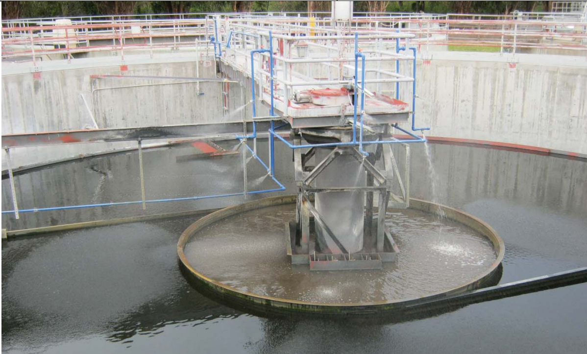
Secondary Clarifier Center Structure
