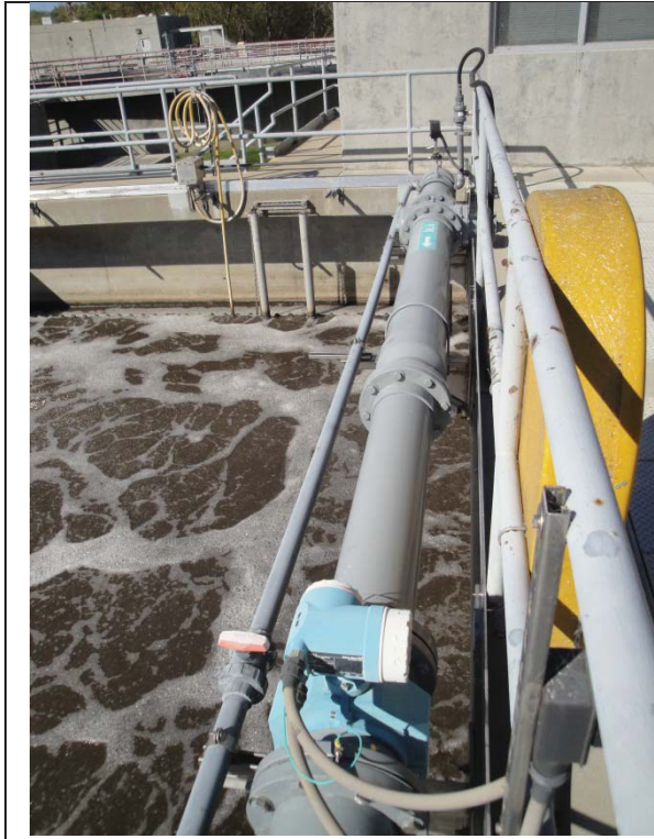
PVC Mixed Liquor Return Piping and Flowmeter
