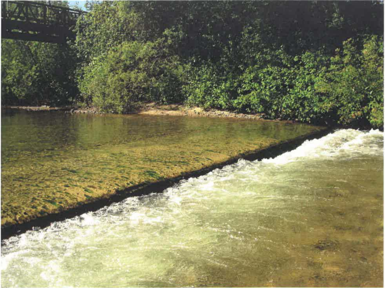
CAWD pipe crossing under Carmel River
