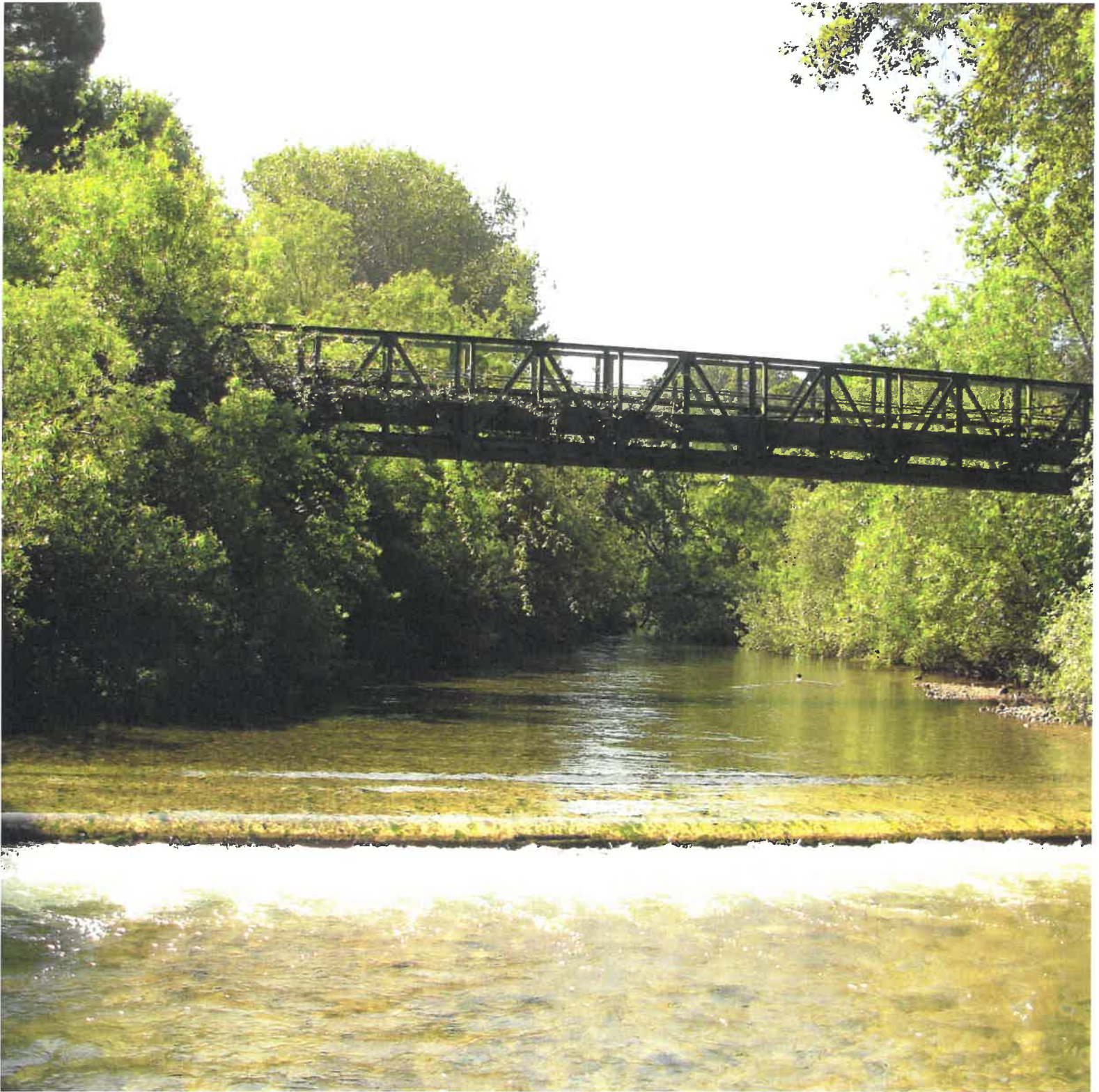
Carmel River Pipe Crossing
