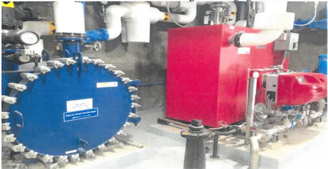
Digester Control Building #1 – Spiral Heater and Boiler
