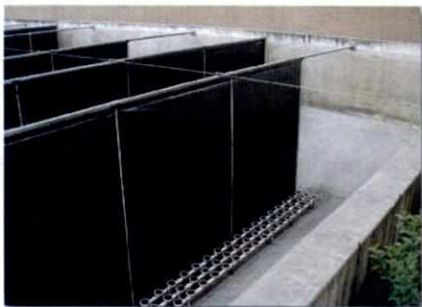
DIRECT FLOW WITH BAFFLES
