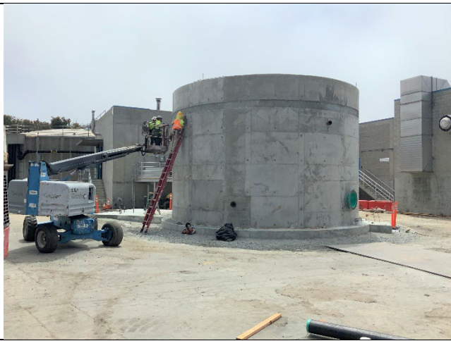
Photo: New Sludge Tank Under Construction
