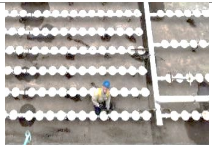
Photo: Existing air diffuser system
