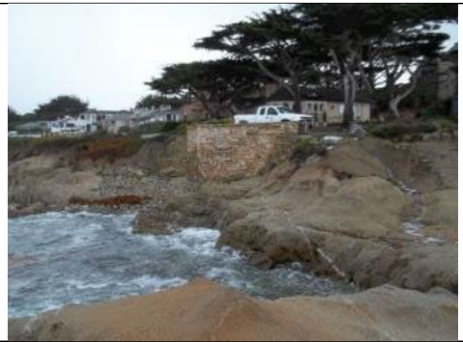
Photo: Looking at Pump Station Exterior
