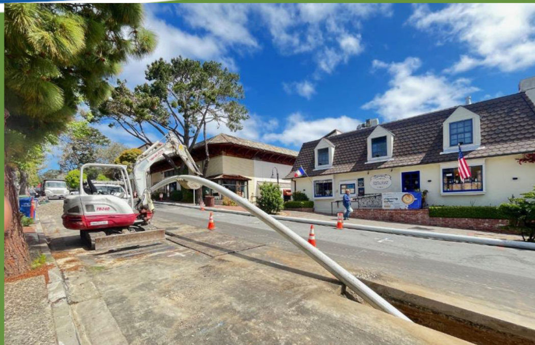
Photo: Pipe bursting on Mission St.
