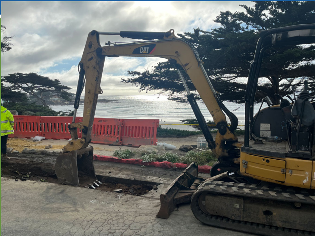
Photo: Digging trench on Scenic Rd.
