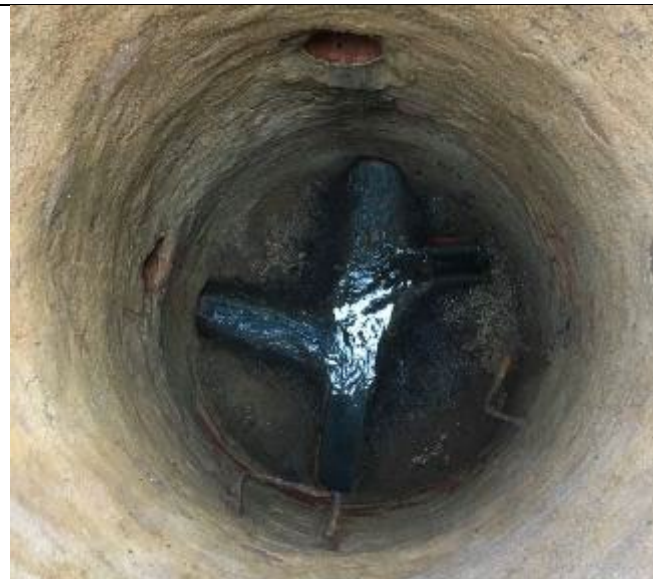
Photo: Inside of Sewer Manhole
