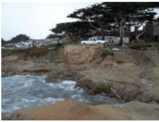
Photo: Pump Station Exterior
