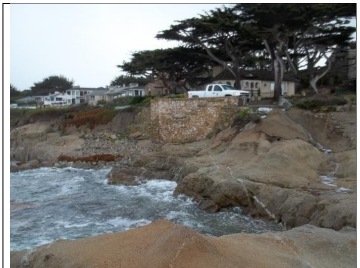
Photo: Looking at Pump Station Exterior
