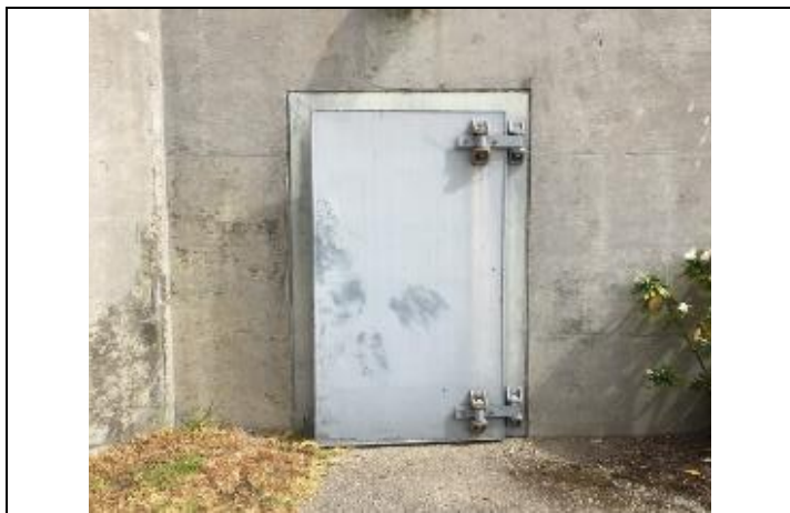
Photo: Old Flood Door in Headworks Basement
