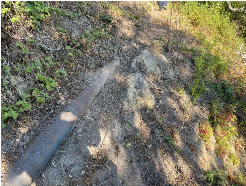
Figure 1: Limited cover, narrow access, steep slopes
