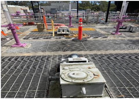
Photo: Existing Coagulation/Flocculation System and Sand Filters
