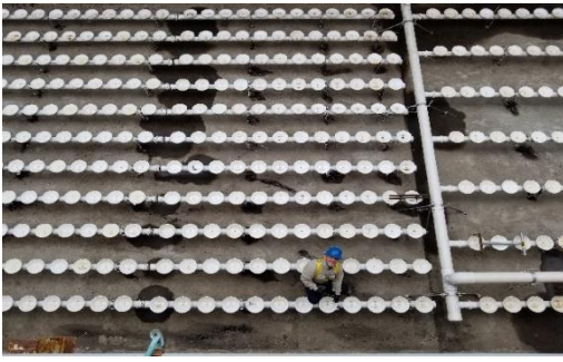
Photo: Existing air diffuser system
