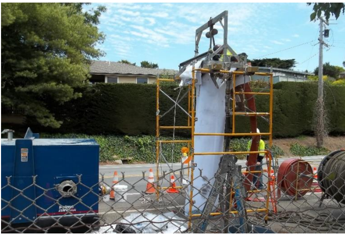
Photo: View CIPP Liner being installed
