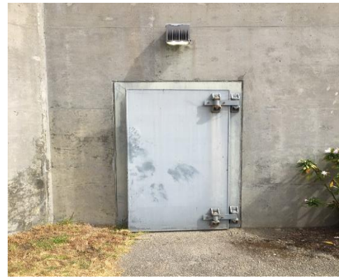
Photo: Old Flood Door in Headworks Basement
