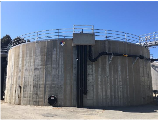
Photo: Digester No. 1
