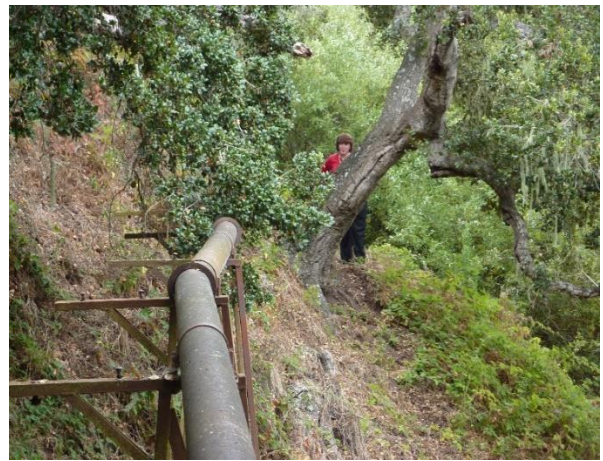
Photo: View gravity pipe in Carmel easement
