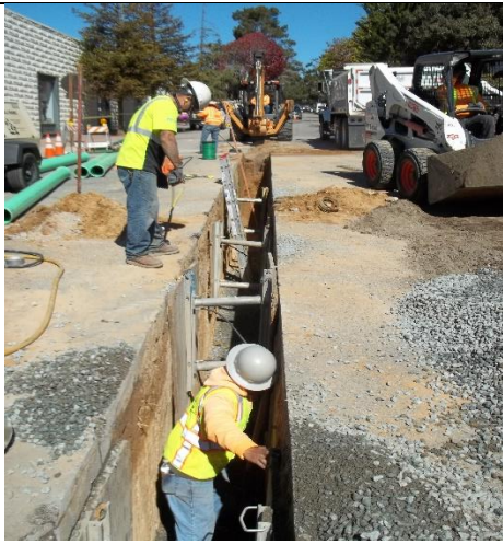
Photo: View of sewer line being replaced
