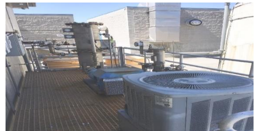
Photo: Existing Gas Conditioning System
