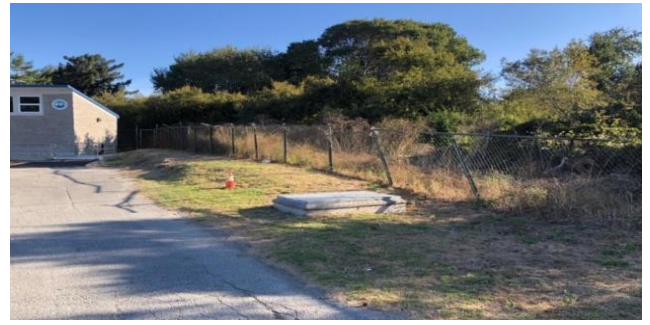
Photo: Eastern side of Perimeter Fence
